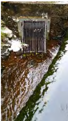
Figure 1: Intake at Haipuaena stream
