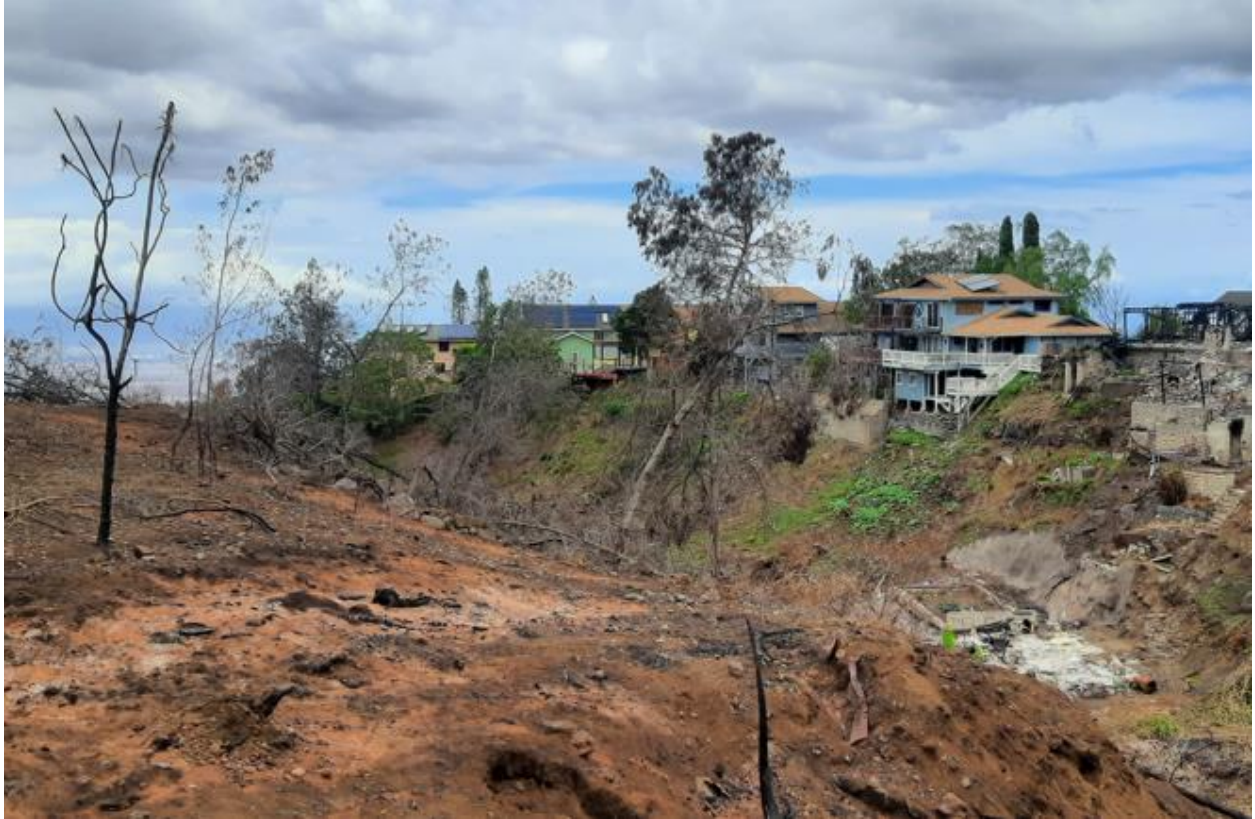
Several of about 25 houses at risk of foundation erosion along Pulehu gulch
