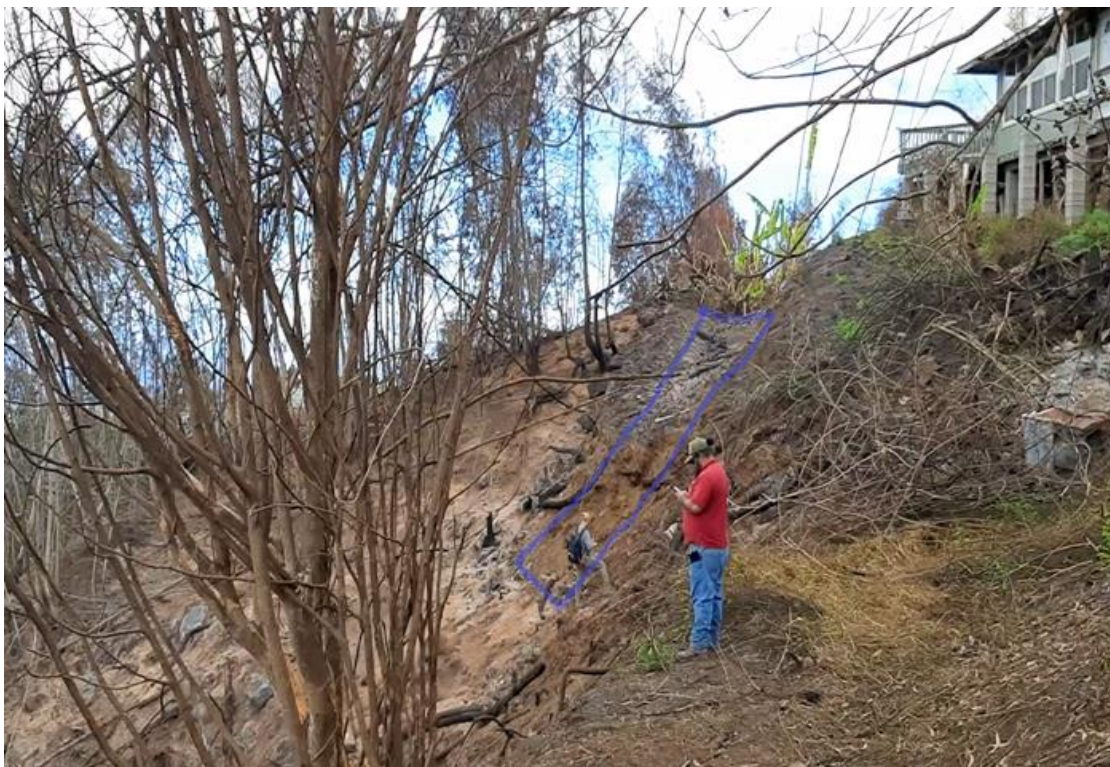
Site of proposed gabion mattress to control erosion (blue outline)
